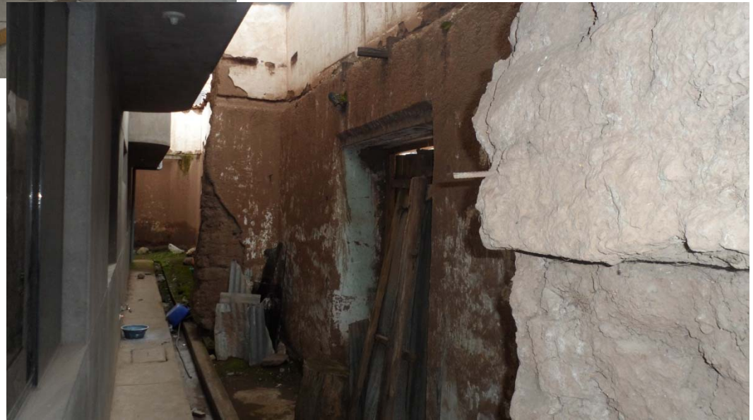
Outer wall before and the first step
